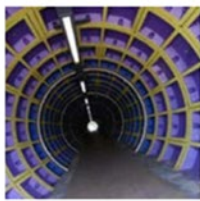
Circular tunnel forming rings
