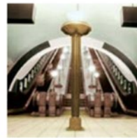
SOUTHGATE STATION Escalators
