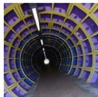
Circular tunnel forming rings
