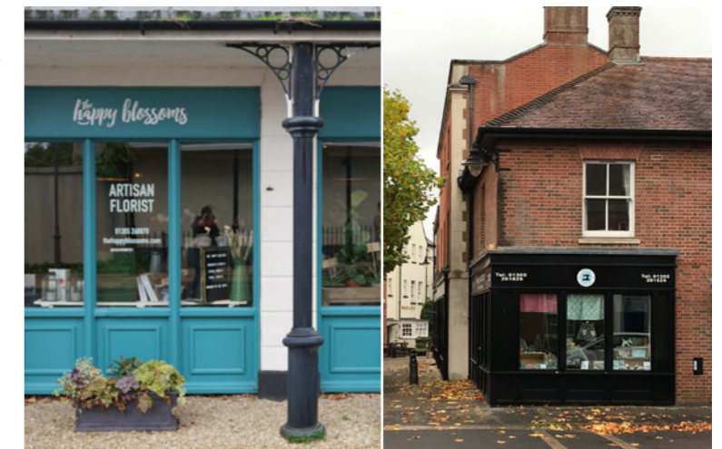
Scattered workshop units on ground floor are successful independent businesses and provide a different offer to Dorchester high street comparison retailing.
