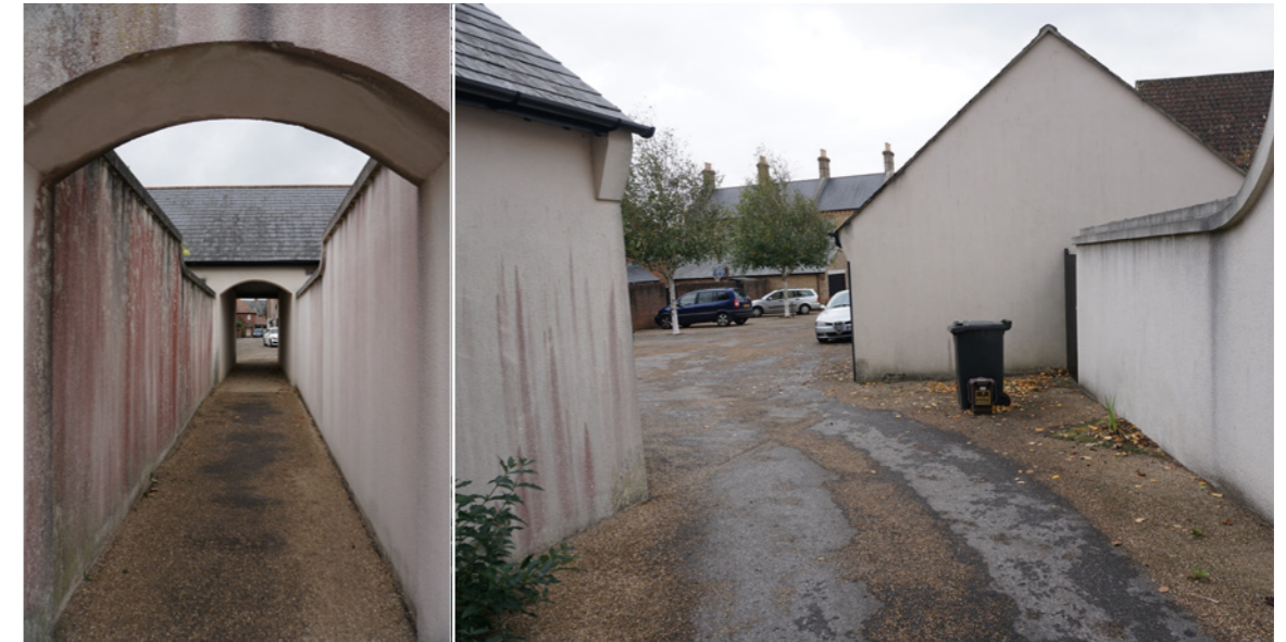
Organic medieval masterplan with parking garages in courtyards results in many external spaces and paths criss-crossing the housing. Not all of these have apparent use and some lack overlooking as they are flanked with blank walls.
