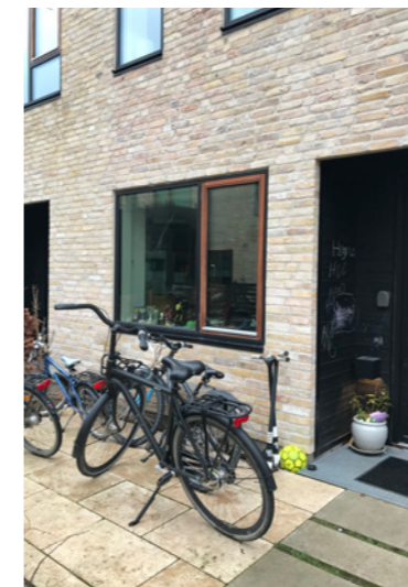
Semi-private entrances to the houses used for bike parking. Chalkboard in entrance to house - personalisation.
